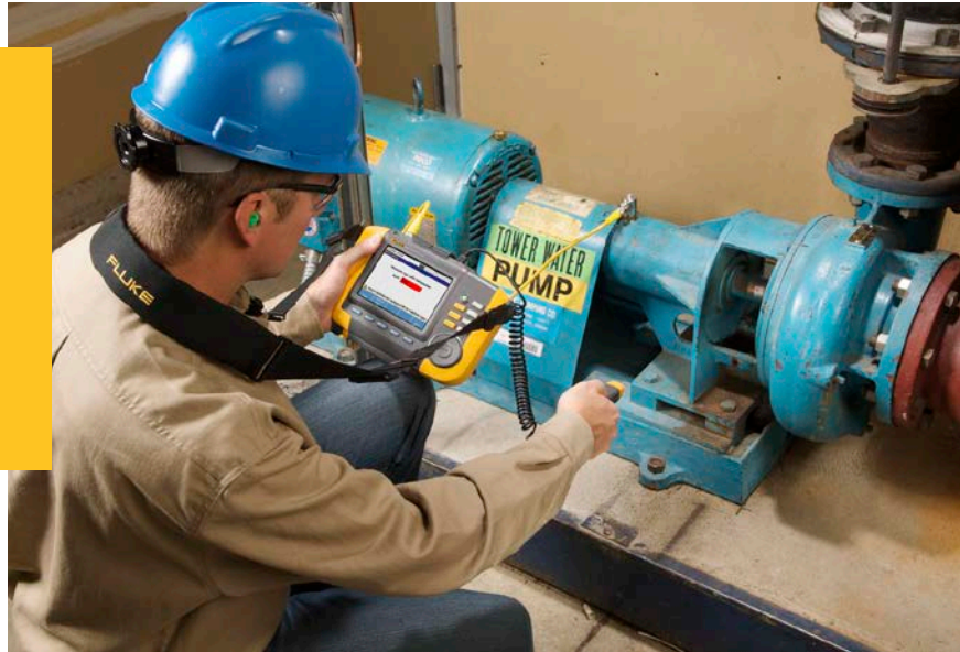
Understanding vibration analysis can change a “run to failure” system to a condition-based, proactive maintenance program.
